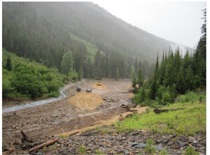
**Snowshoe Crk Project:** Upper photos depict conditions in the valley bottom prior to construction. Note the toxic mine and mill tailings in the creek bottom. Lower photos show current construction activities after tailings have been removed and stream bed is being reconstructed. Tailings were removed and encapsulated in the repository facility shown on the cover of this report.
